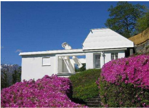
Fig. 2. IRSOL Observatory. In the left side of the building there is the observing room, while the spectrograph room is in the underground. All is white painted with titanium dioxide.
