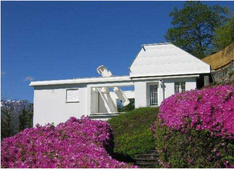
Fig. 1. IRSOL Observatory. In the left part of the building there is the observing room, while the spectrograph room is underground. All is painted white with titanium dioxide. The institute is located 500 m above sea-level, above the city of Locarno, Switzerland.
